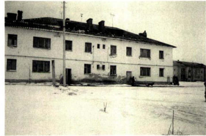
29. At Verchnyua Troitsa, one of the new village’s two-story houses, each containing sixteen flats
