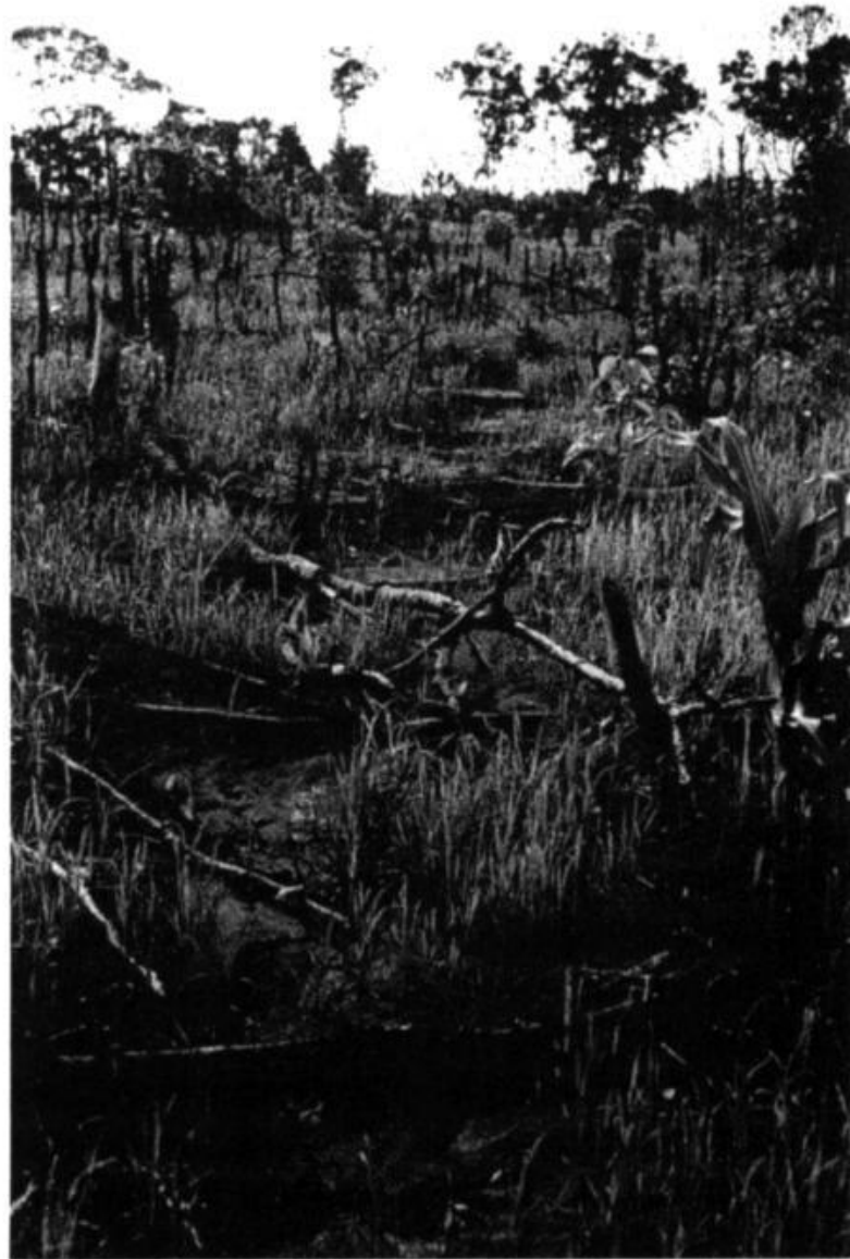
35. Construction of stick bunds across incipient gullies in a Sierra Leone rice field
