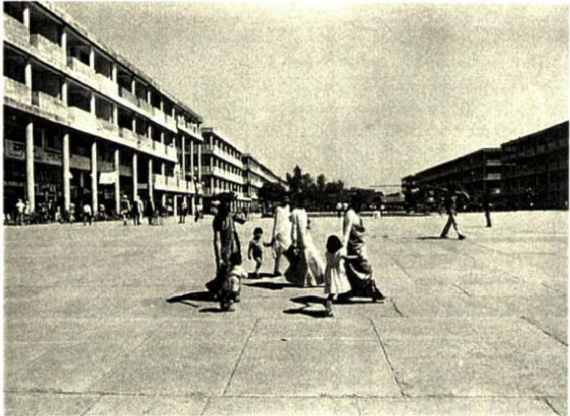
27. The chowk, or piazza, that Le Corbusier designed for Chandigarh's city center
