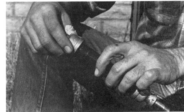
First, screw the reducers on the ends of the pipe nipple.
