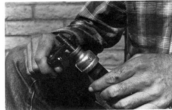
Then, using vise-grips, screw the 1/4 inch nipple into one of the reducers (as tightly as possible).
