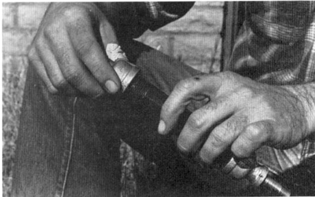
First, screw the reducers on the ends of the pipe nipple.
